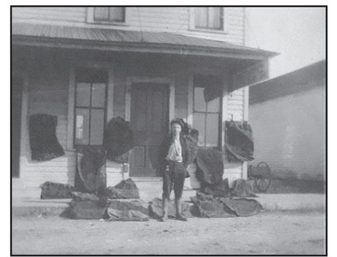
The Post Master often had to dry the mail bags on the front porch of the building.
